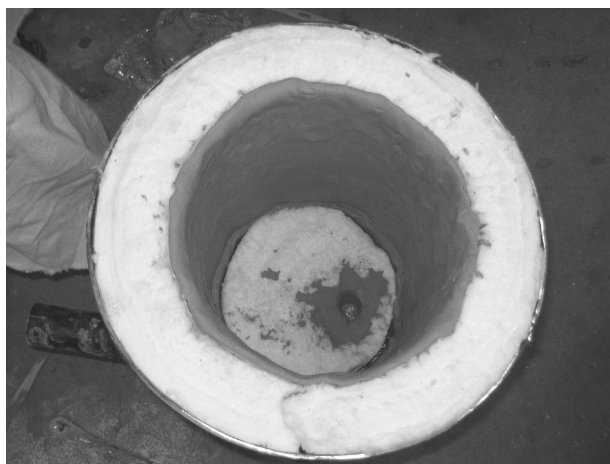
Figure VI-6: Hotface sidewall installed in the furnace
