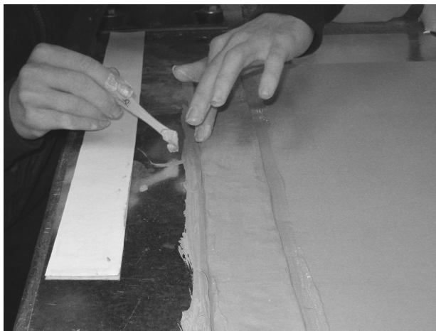
Figure VI-5: Blending floor support strip into hotface sidewall
